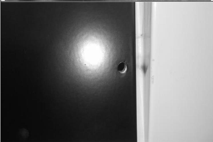
39. When the alignment is achieved drill  $\text{Ø}6.5\text{mm}$  hole through tub face. Remove temporary fasteners holding beaver panel in place. De-bur the hole to remove all sharp edges.
