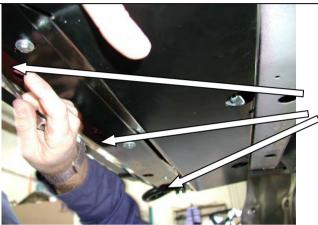
35. Fit three M8 cage nuts to square holes inside the bar. Bolt the deflector to the bar using M8 bolts, large M8 flat washers and spring washers.
